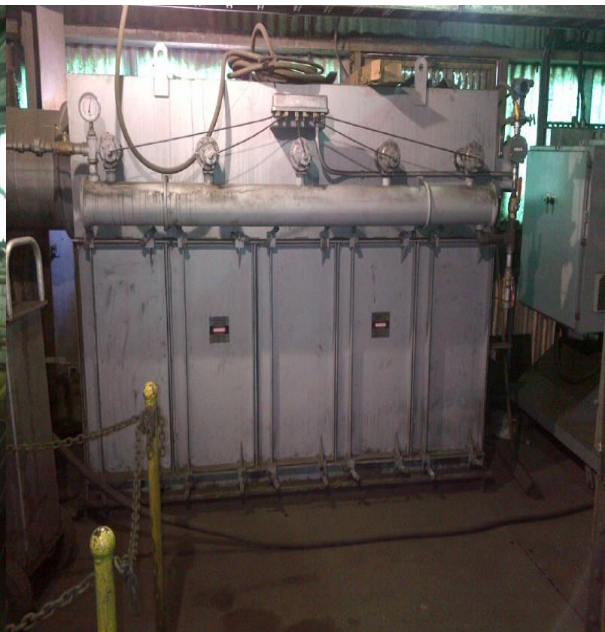
Figure 18. - New Bin Vent on the Matte Silo Matte (2014)
